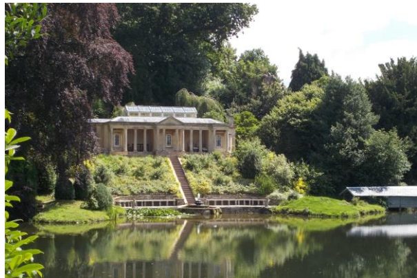
The Temple at Stancombe Park
